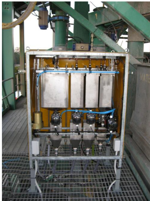
HMT Admixture scale (Cladding removed)
